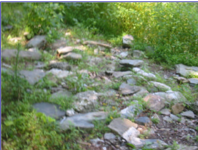
Figure 9. Rip-rap slope protection along the upstream slope
