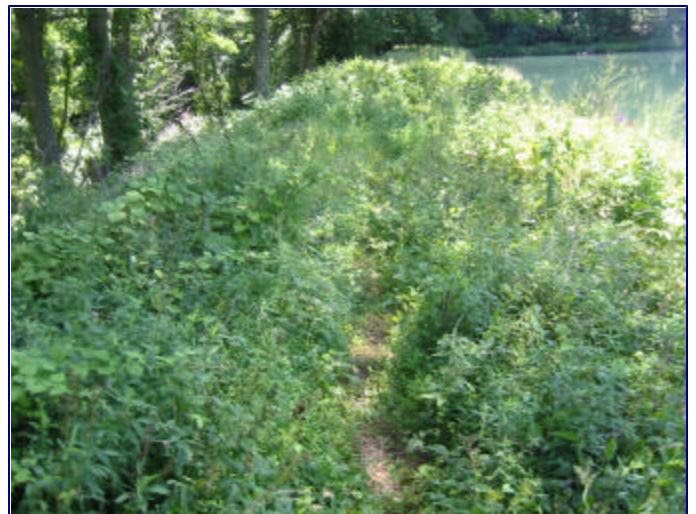
Figure 10. Looking south along dam crest
